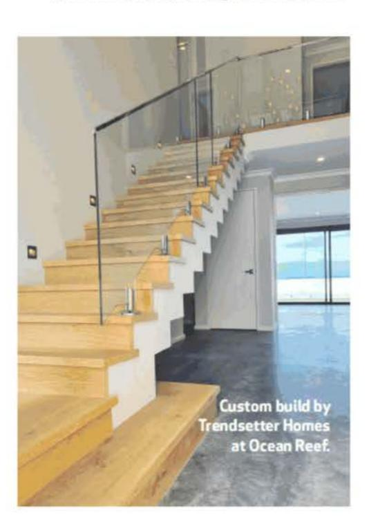
"Unlike polished concrete, burnished concrete is created without the use of grinding," she said. "Shortly after pouring, a trowel machine equipped with steel trowel blades is used to further smooth and compact the surface.
